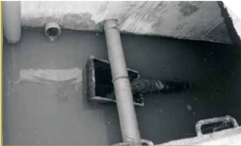
Feeding tank and mechanism - Optimum water level in the tank, just going to fill in the bucket (Shrestha, R.R., 1999)
