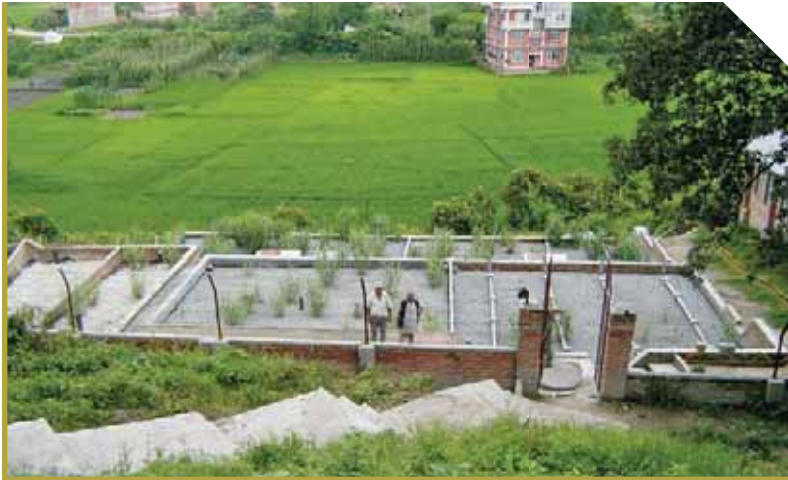
A view of the constructed wetland after completion
