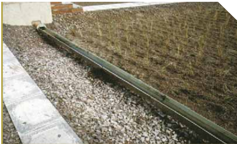
Channel inlet (Cooper et al. , 1996)
