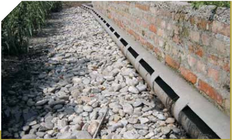
A view of clogging of perforations due to sludge drift from primary treatment
