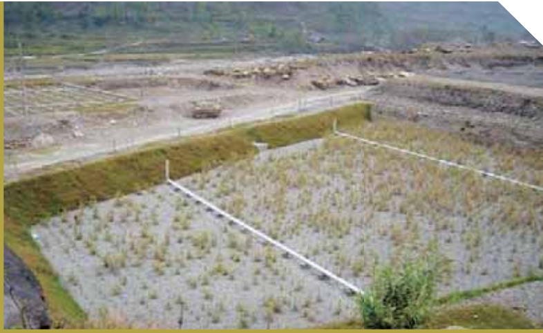
Horizontal flow constructed wetland (Shrestha R.R.)
