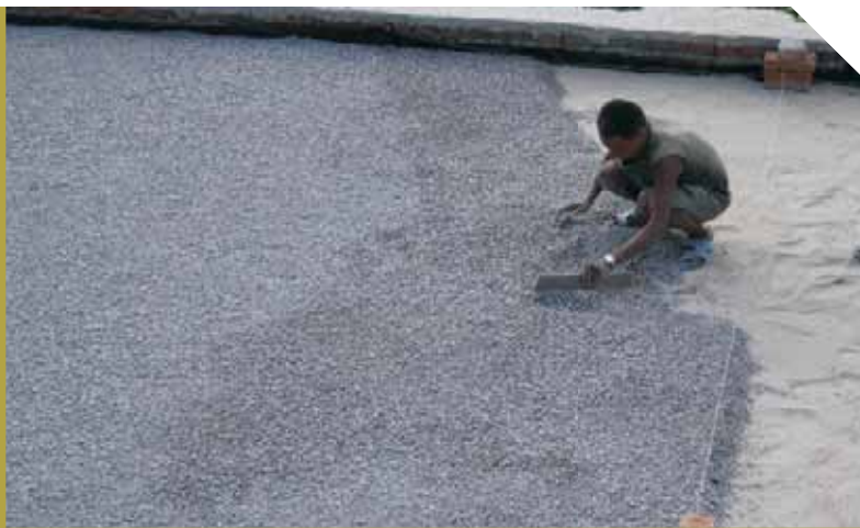
Filling of substrate (protection layer) in vertical flow CW
