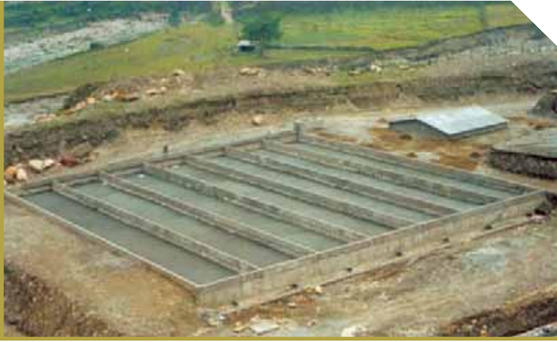
Sludge drying bed (Shrestha R.R.)
