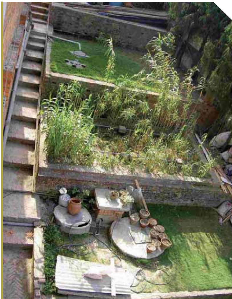
Constructed wetland at ENPHO PLATE 39
